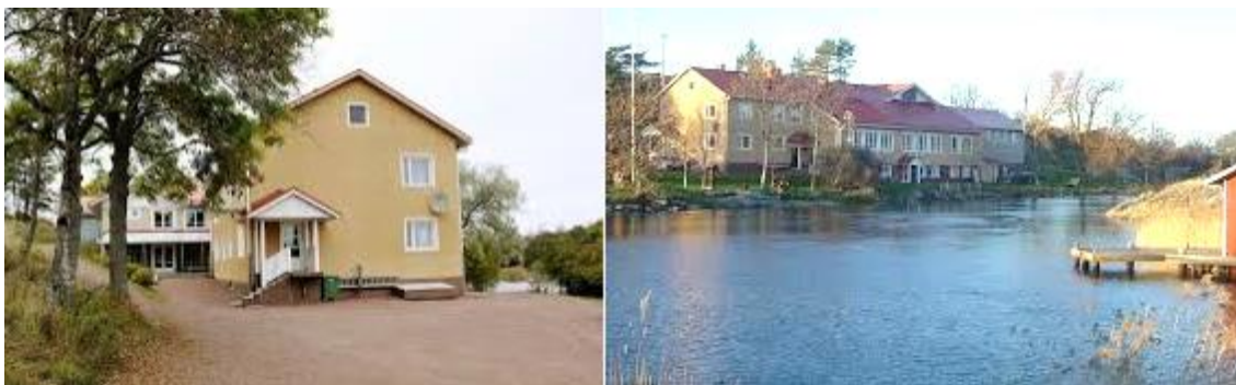
Figure 3: Pictures of the Karlby school building
