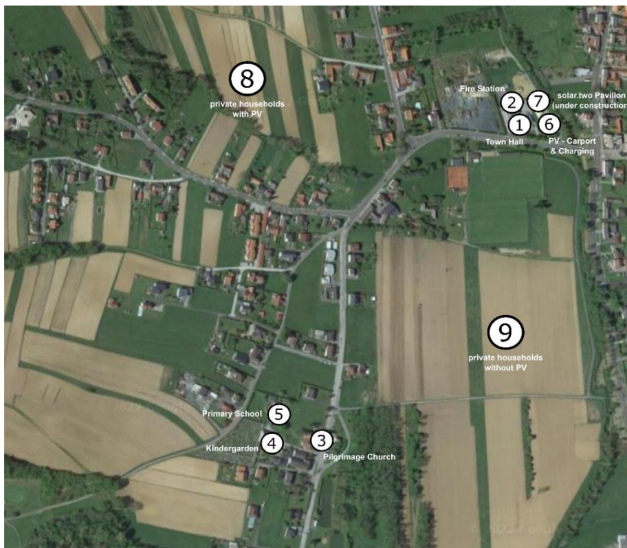
Figure 14: Bird view of the municipality Ollersdorf with the participating municipal buildings
