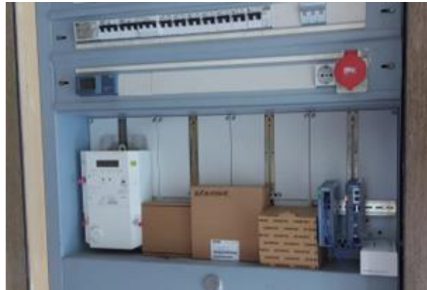
Figure 18: Installation of the smart ICT in Ollersdorf
