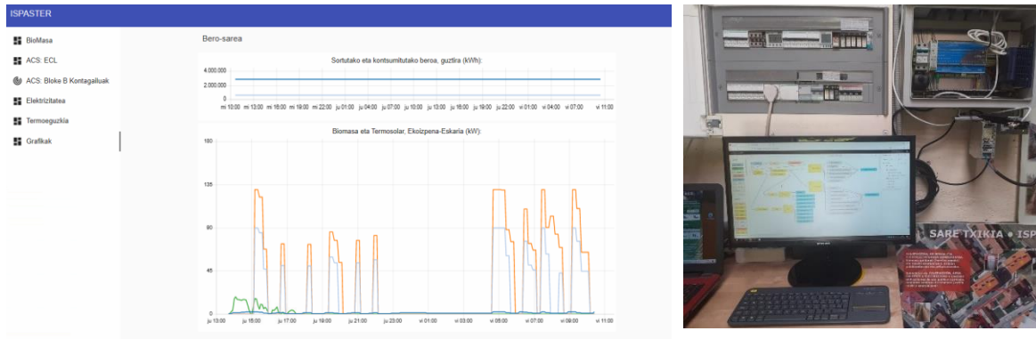
Figure 17: New SCADA data-communication platform
